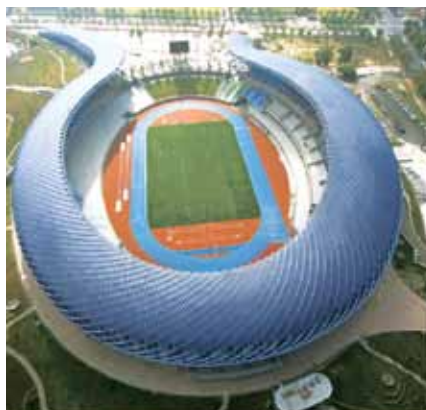
Saddle-shaped solar-panel roof of 2009 World Games Stadium, Kaohsiung, Taiwan (Courtesy Delta Electronics, Inc.)
