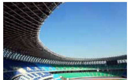
Steel girders of 2009 World Games Stadium, Kaohsiung, Taiwan (Courtesy Toyo Ito Architect).
