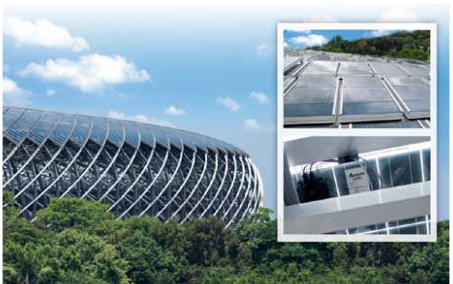
Solar panels of 2009 World Games Stadium, Kaohsiung, Taiwan. (Courtesy Delta Electronics, Inc.)
